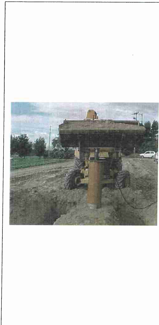
Figure 80: Soil cylinder extraction
